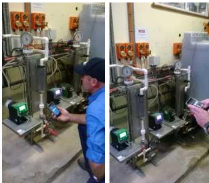
Figure 13: Mobile data collection – an example of a drop test being conducted and the data recorded on-site
