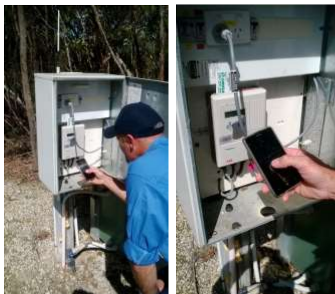
Figure 12: Mobile data collection – an example of cross-check flow meter readings being recorded on-site.
